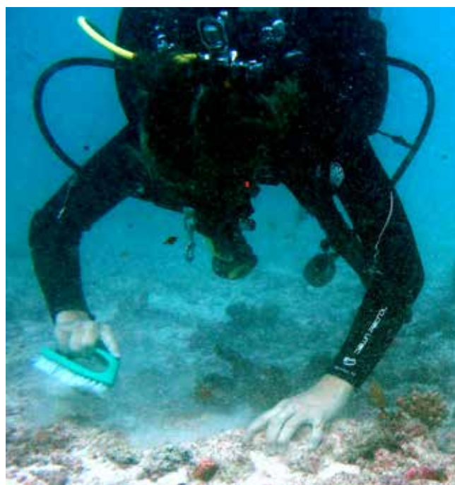
Figure 40 Ensuring areas of suitable hard substrate are adequately cleaned prior to transplanting with cement.
